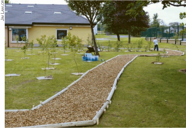
A low-maintenance path with chipped bark surfacing meanders through a newly planted school woodland.
